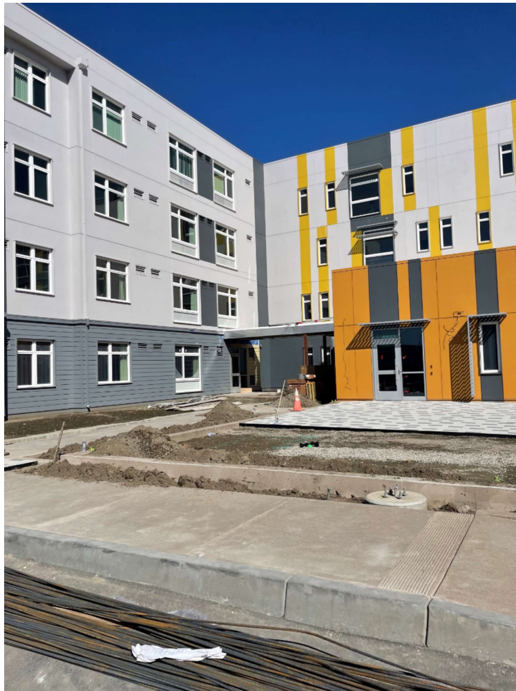
Exterior courtyard cement pours, pathways, pavers and bioretention areas were installed.
