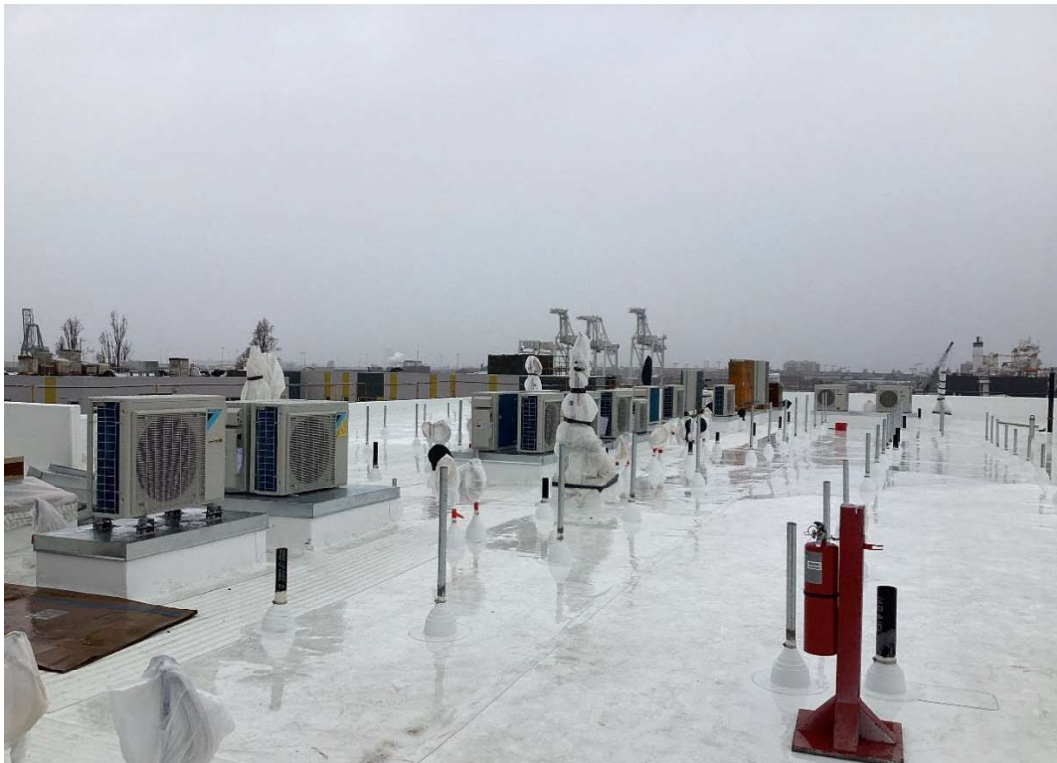
Figure 8: Installation of the heat pumps
