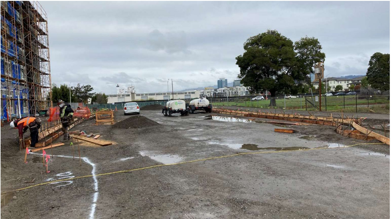
Form work for new curb and gutter at the new Mabuhay Street looking north towards Mosley Ave.
