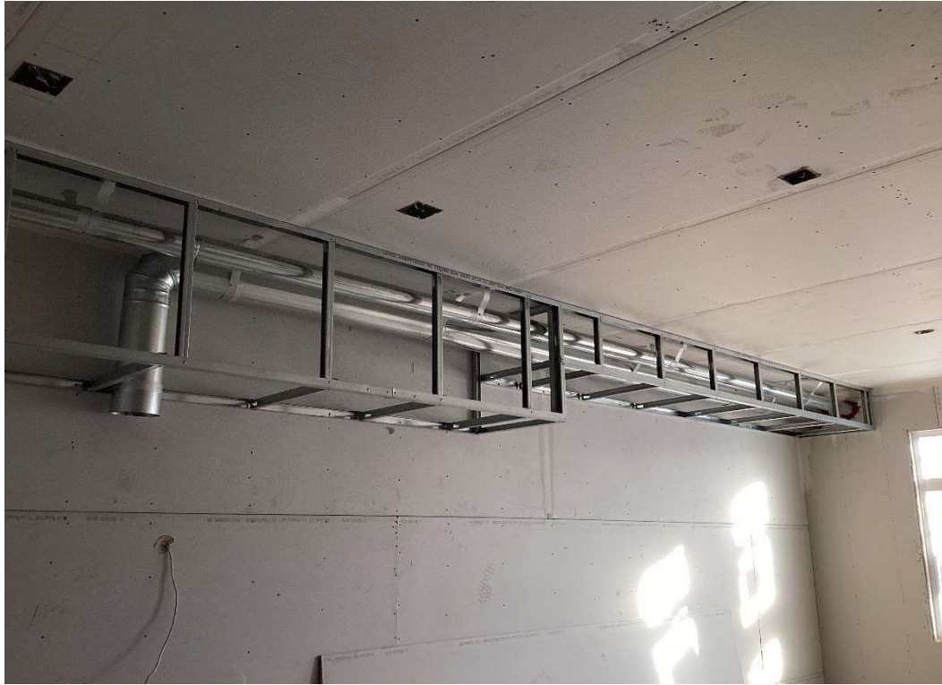
Figure 7: Completion of MEP Installation at units
