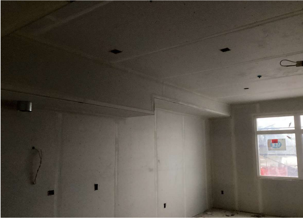
Figure 5: Completion of drywall installation at units
