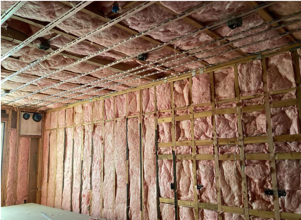
Figure 6: Installation of insulation at units
