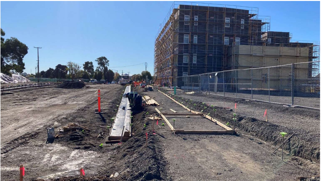
New curb and gutter at the new Mabuhay Street looking south from Mosley Ave, along Estuary II site and Linnet Corner on the right of the photo.
