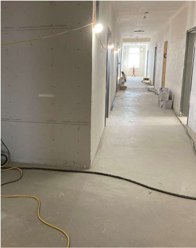
Drywall, tape, texture, and painting in the corridors.
