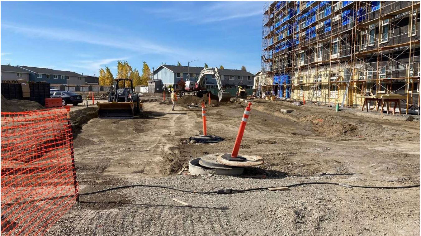
Ongoing grading at the realignment section of Lakehurst Circle, adjacent to Linnet Corner.
