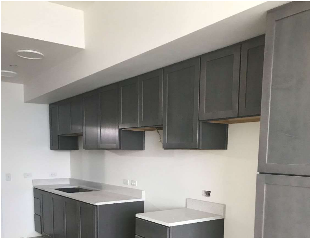
Figure 6: Cabinet installation at level 1
