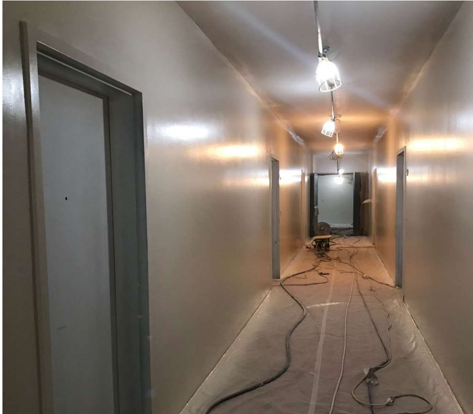
Figure 7: Texture and Paint at level 4
