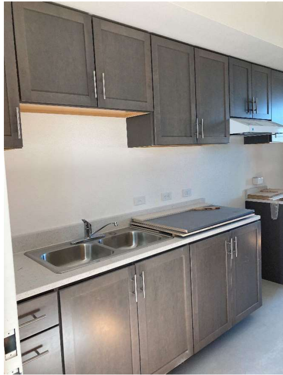
Kitchen faucets and cabinets installed.
