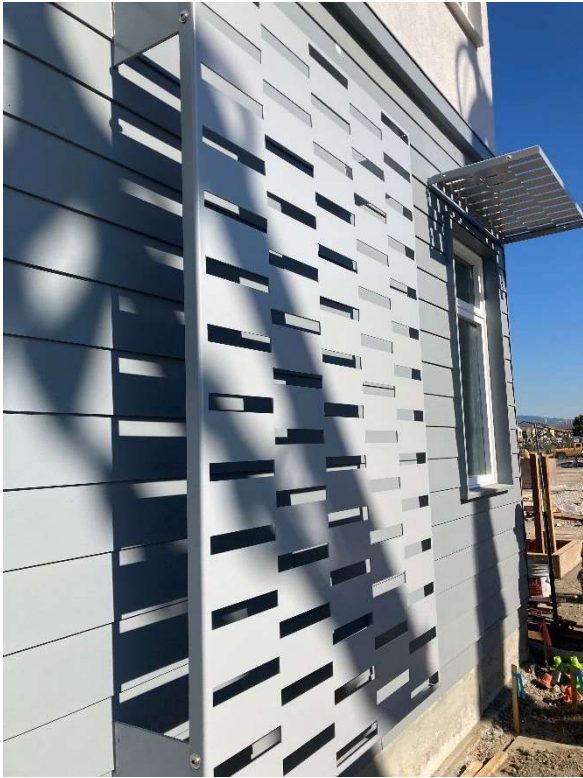
Metal sunshades are installed at the building
