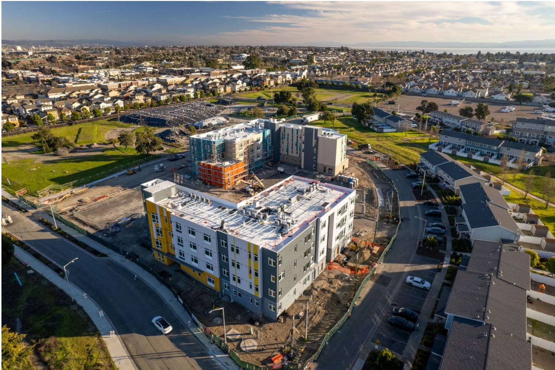
Aerial photo looking south showing the northern and western elevation exterior walls.
