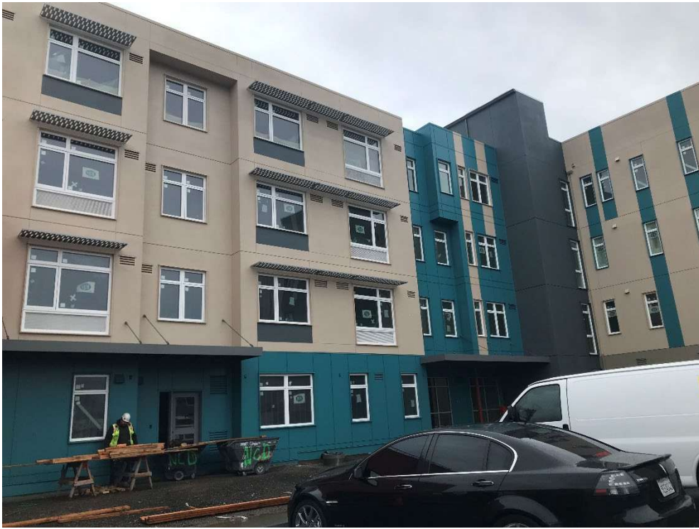
Figure 5: Completion of exterior paint at courtyard elevation
