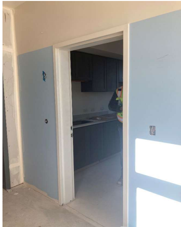
Painting on all floors – 2 nd floor hallway
