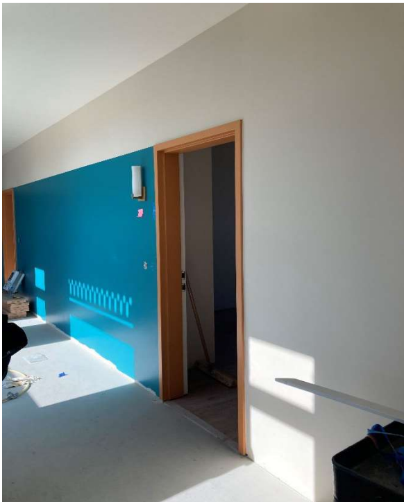
Painting on all floors – 4 th floor hallway
