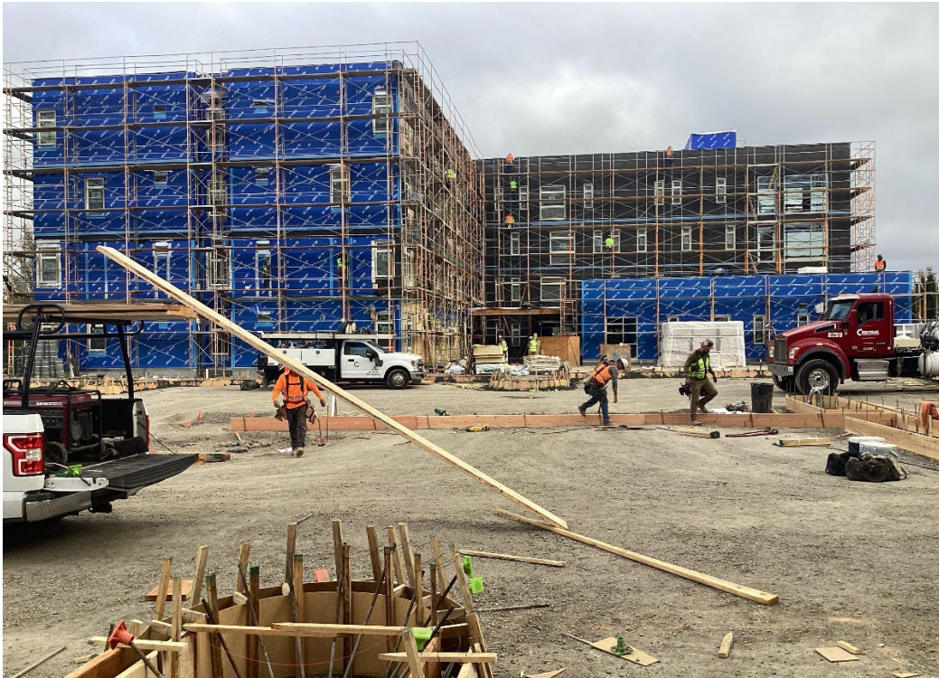
Figure 6: View of north courtyard elevation
