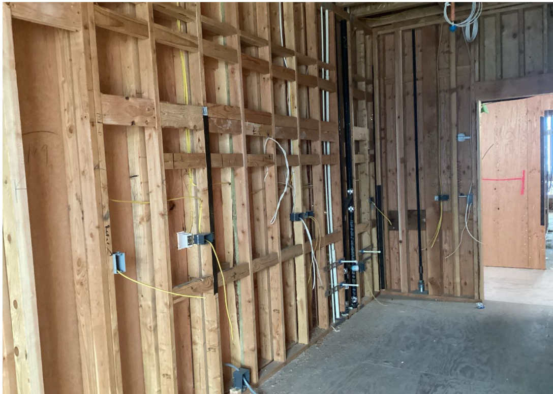
Figure 8: Rough electrical installation
