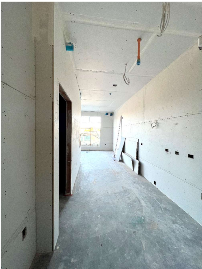
Drywall hung in a studio unit.
