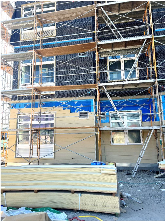
Exterior siding installation on the building elevation.
