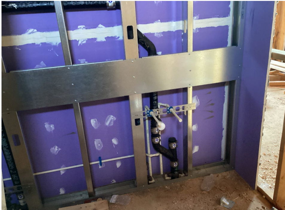
Figure 8: Water Line installation
