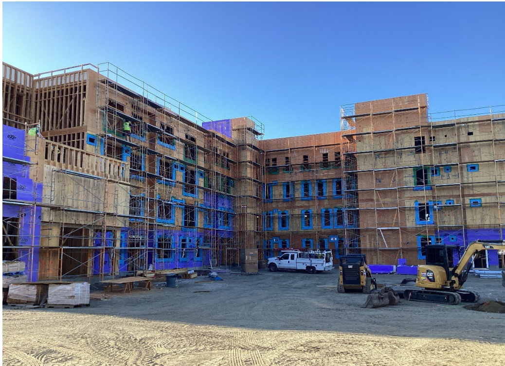
Figure 6: View of north courtyard elevation
