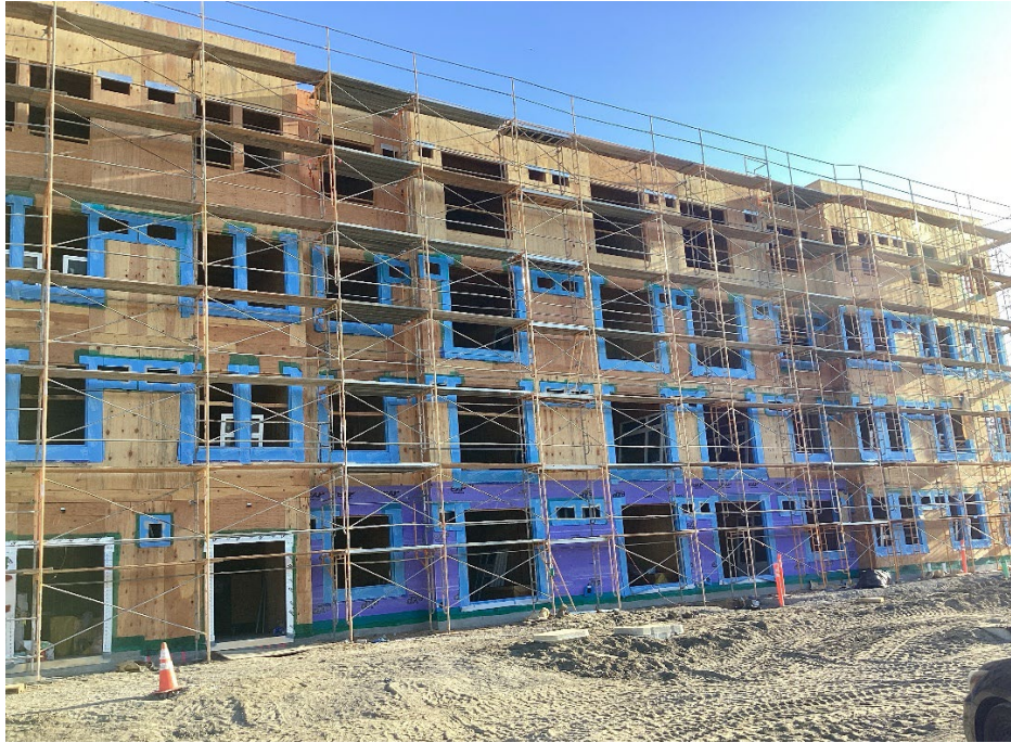
Figure 7: Louver & Window Installation
