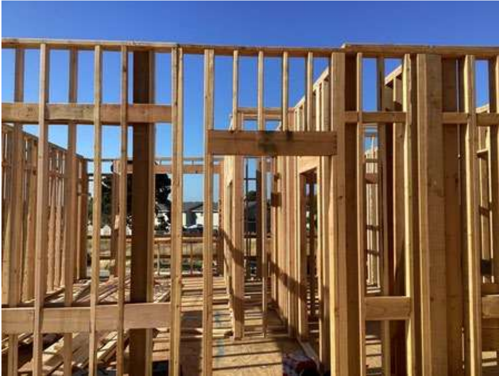
Figure 1: Walls going up at Level 2
