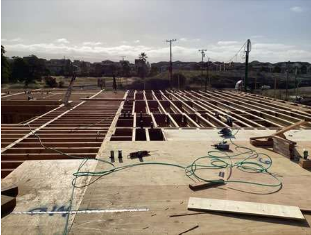
Figure 4: Joist installation at units
