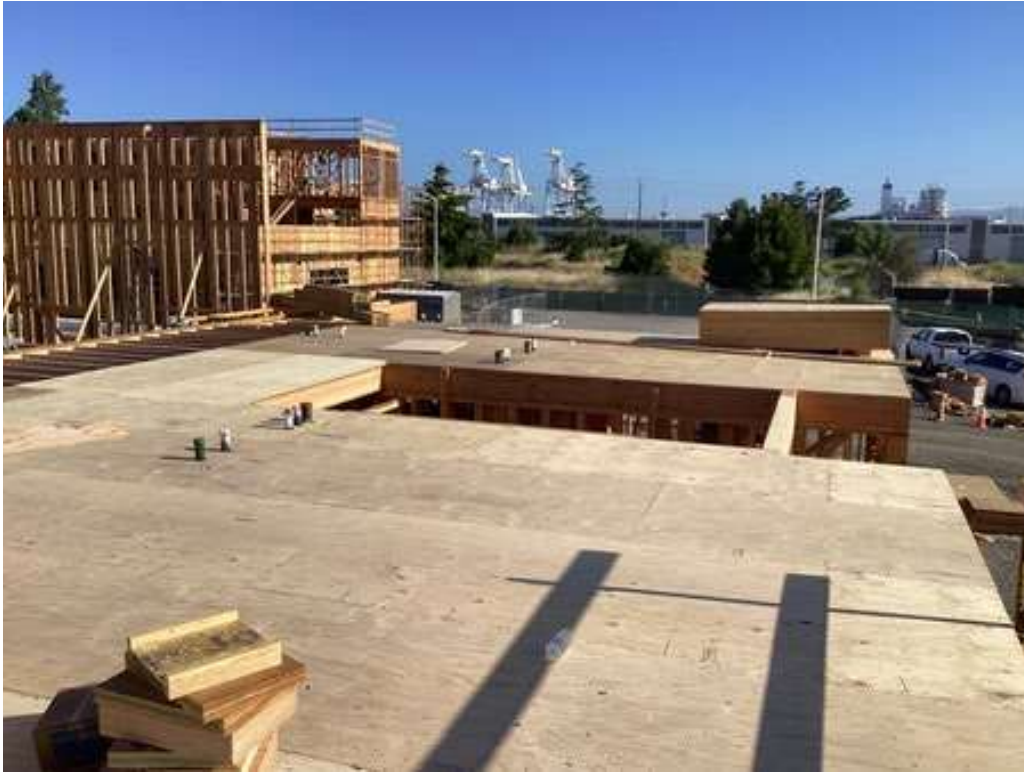
Figure 2: Subfloor Installation at Level 2
