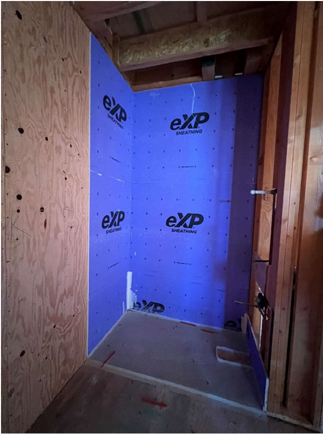
Drywall and gypcrete for the bathtub.
