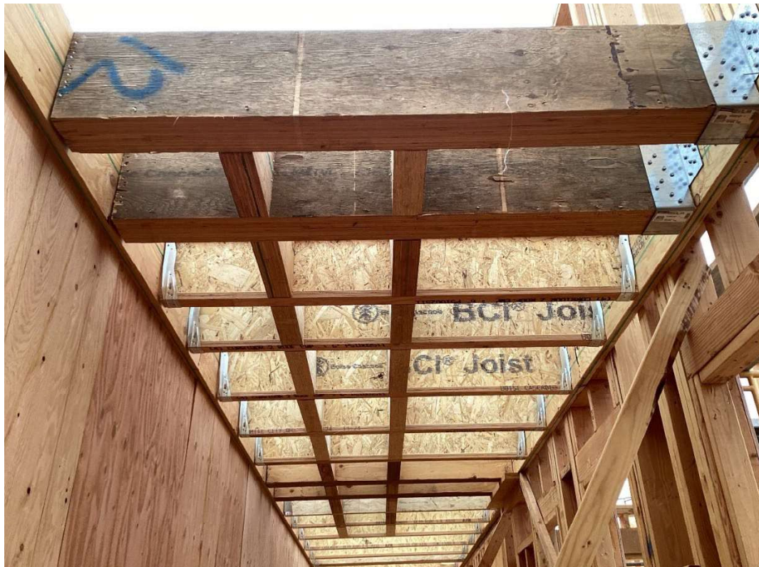
Figure 6: Photo of joists and beam installation
