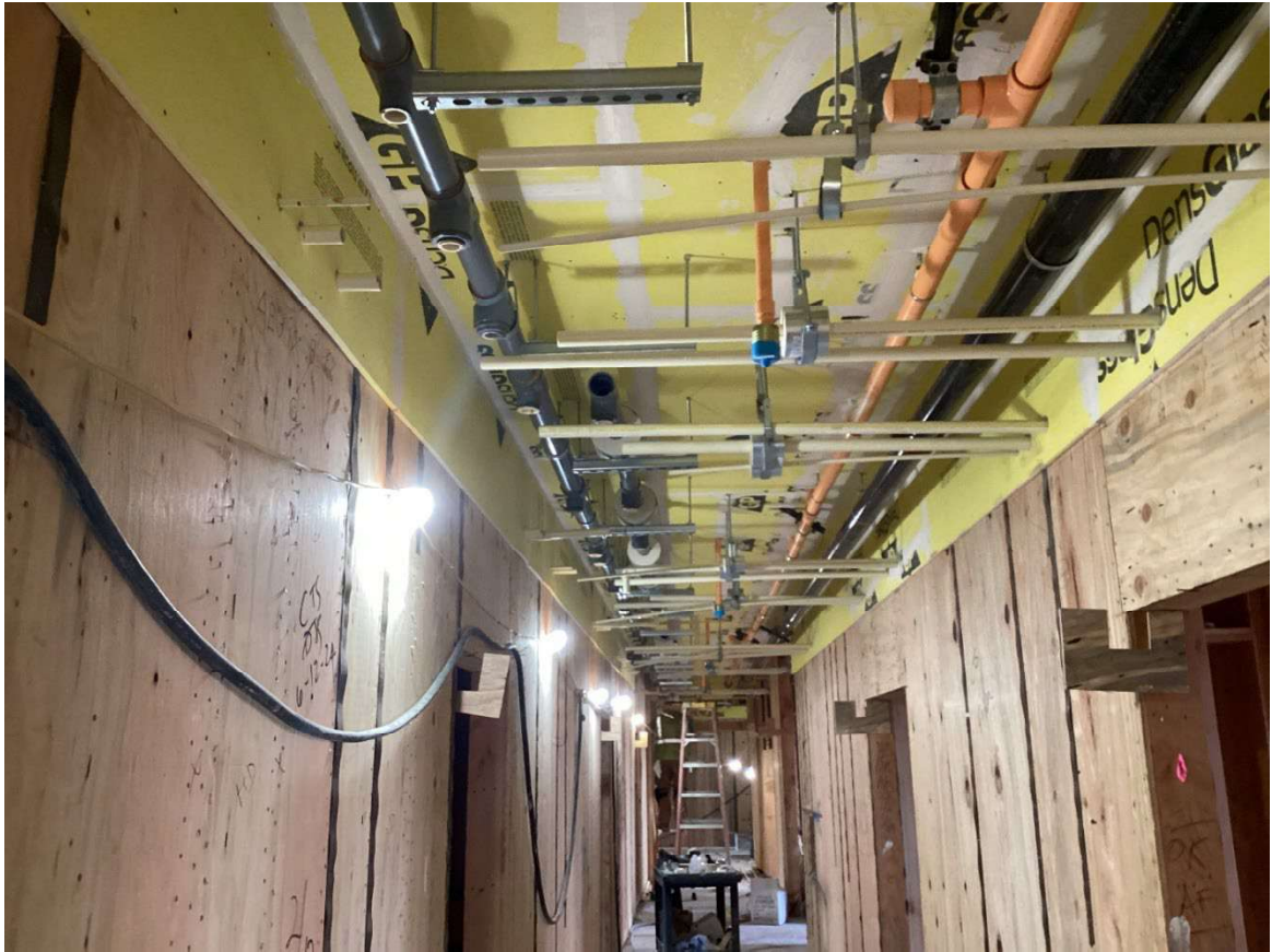
Figure 7: View of water main installation
