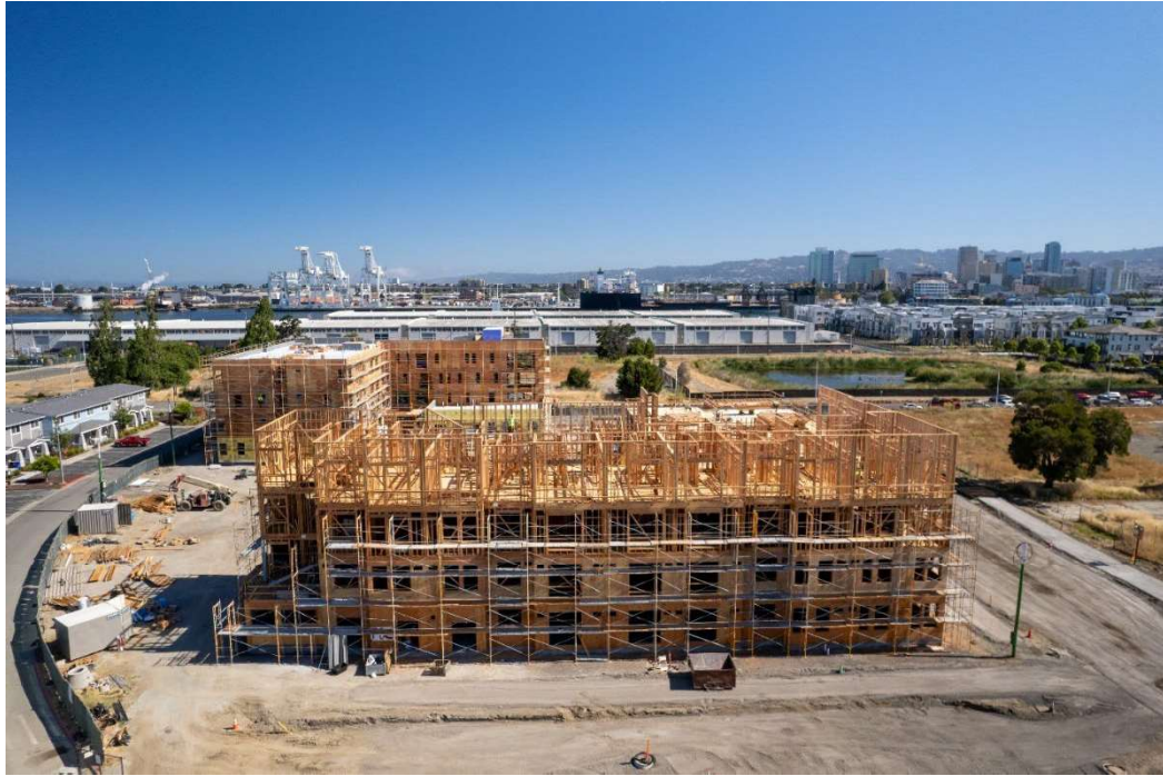
Figure 5: View from Mabuhay Street of framing and scaffolding progress
